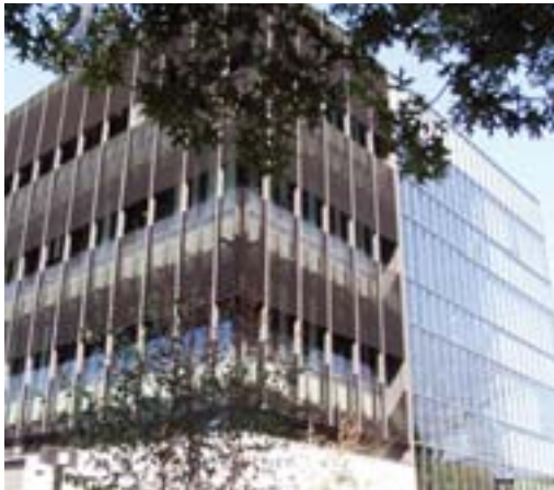
Yale University, New Haven, CT Architect: Kieran Timberlake Associates, LLC
