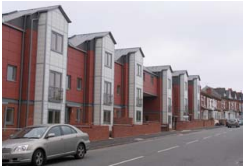
Bearwood Road Apartments, Smethwick, Birmingham, UK Architect: BM3 Architecture
