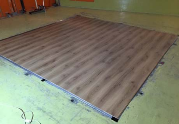
Figure 1: Boards in place on underlay.
