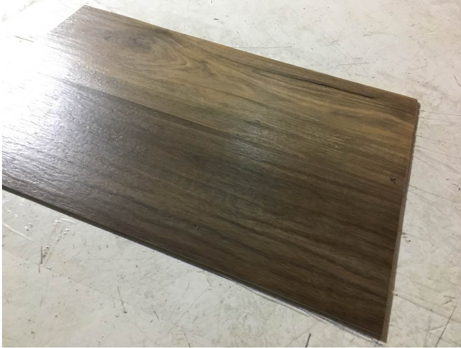
Figure 1: LG Decotile Plus Vinyl flooring adhered to concrete slab
