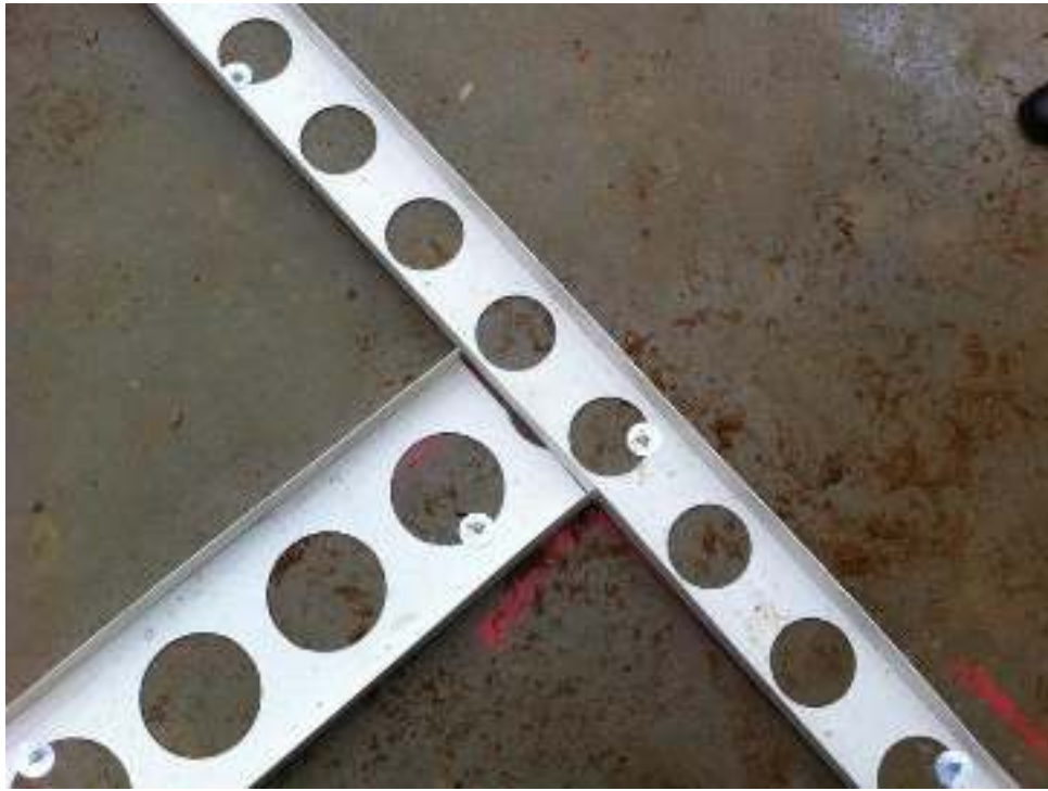
Photo No: 5 Guide Track Placement
